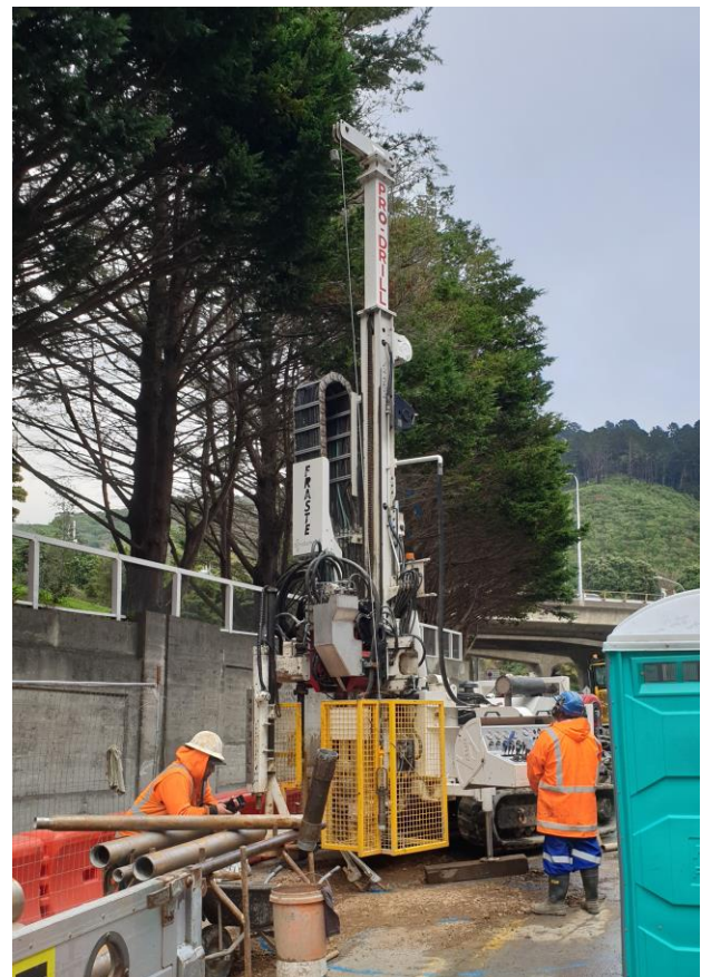
Drilling through the crown of the Interceptor
