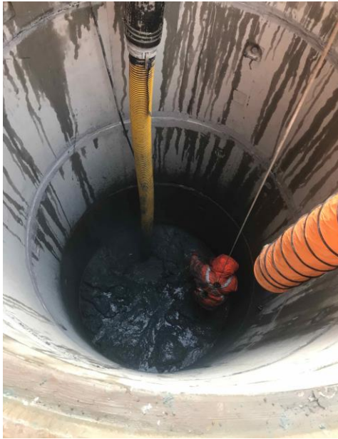
Caisson sinking using hydro-excavation
