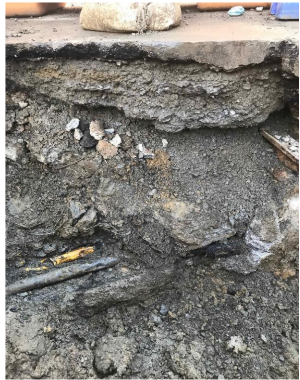
Communications Cables Cast into Concrete Tram Slab and Subbase
