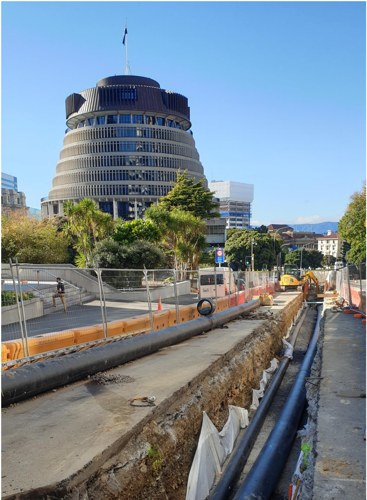
Shared Trenching for the Rising Main and Gravity Main in Bowen St.
