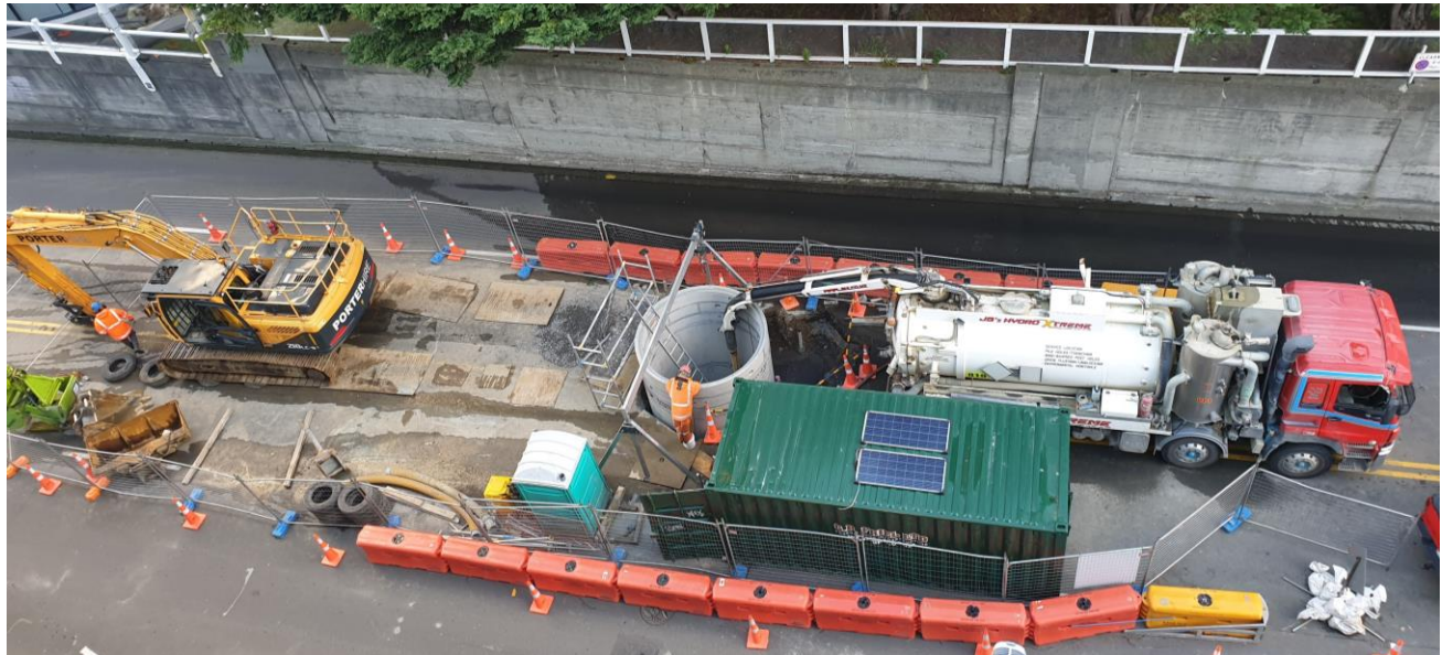
A Birds Eye View of the Interceptor Connection Chamber
