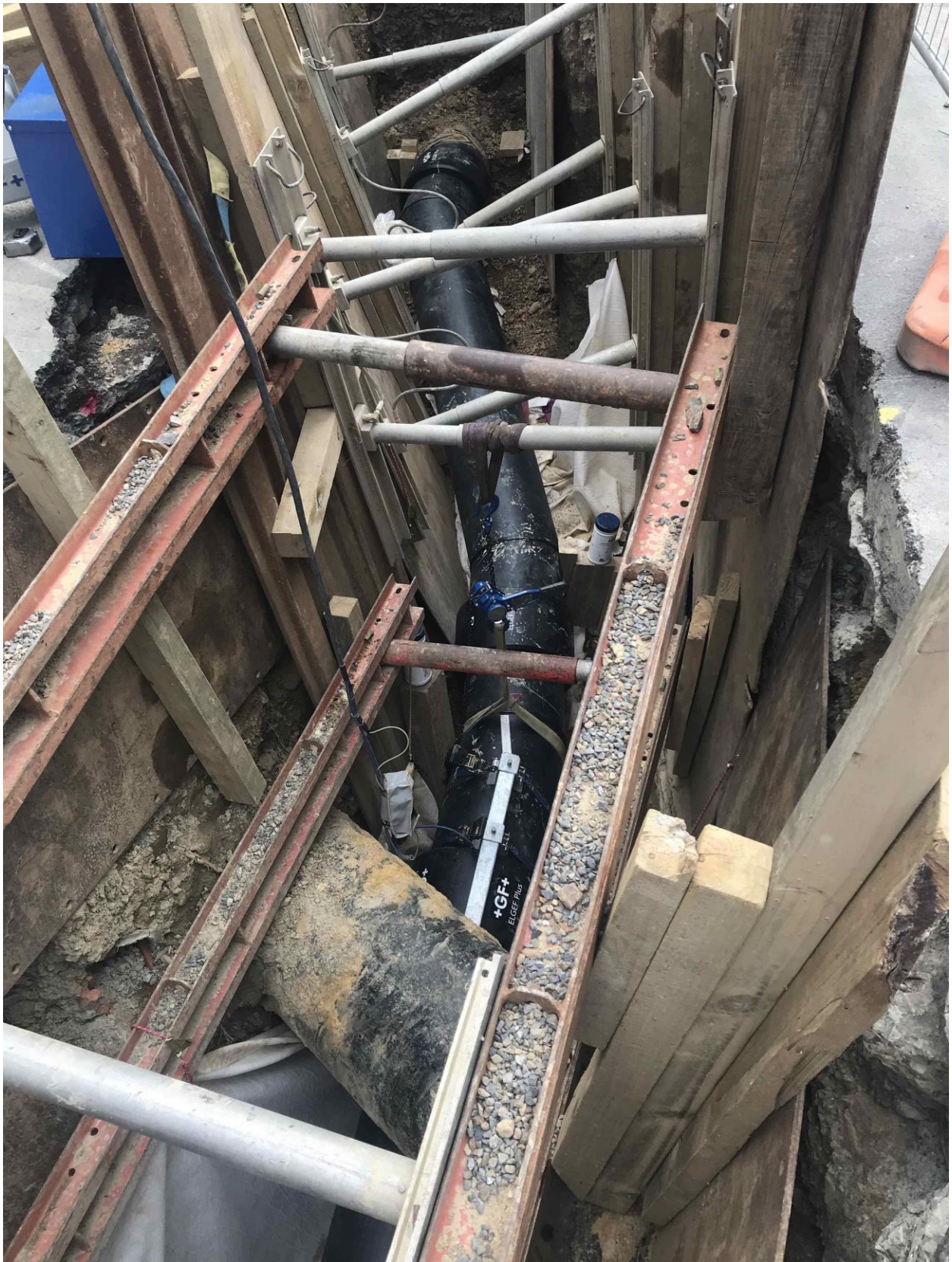
EF Welding around challenging underground services in The Terrace
