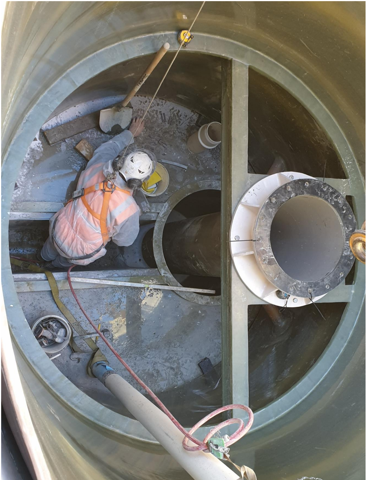
Installation of the FRP liner and drop structure
