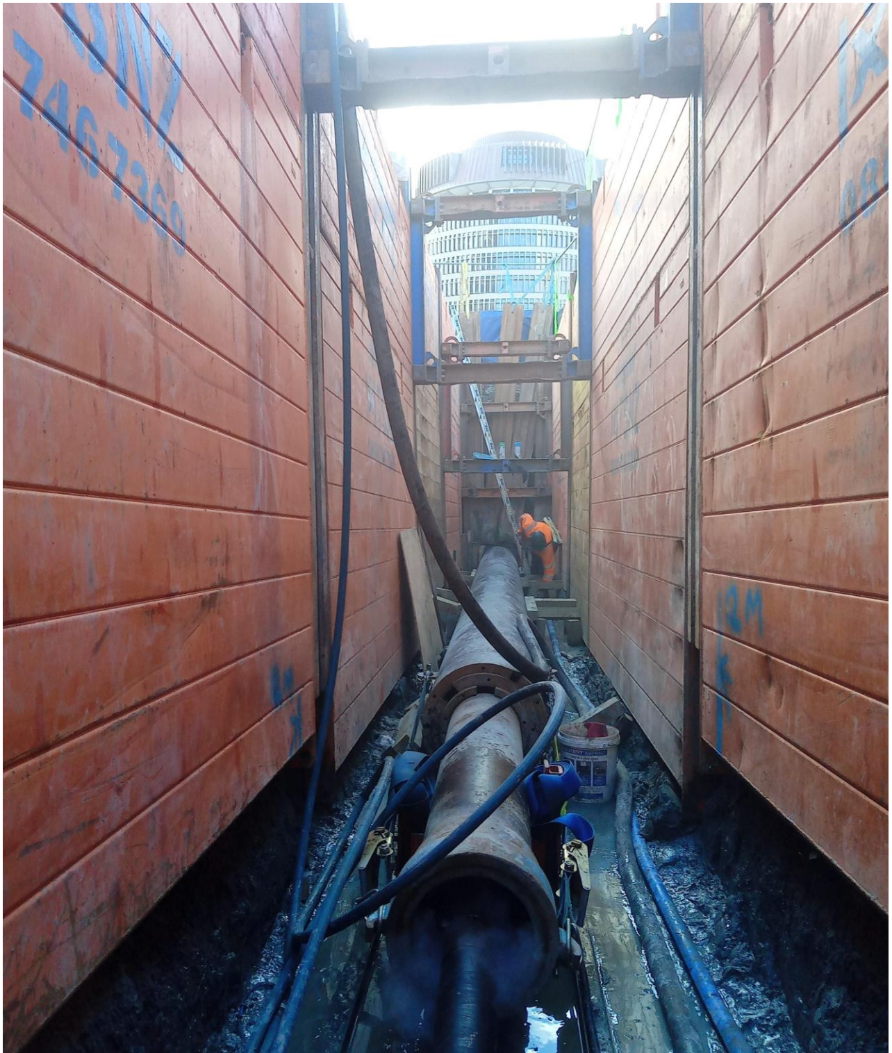
Pipe Ramming under Lambton Quay
