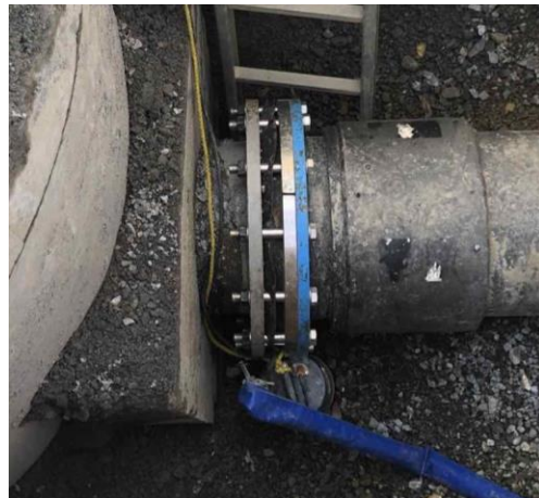
Modified Stub Flange & Backing Ring Arrangement
