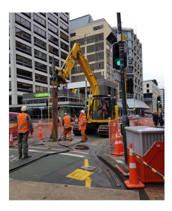
Installation of a deep well using a pneumatic pipe bursting tool – Willeston St/Victoria St Intersection
