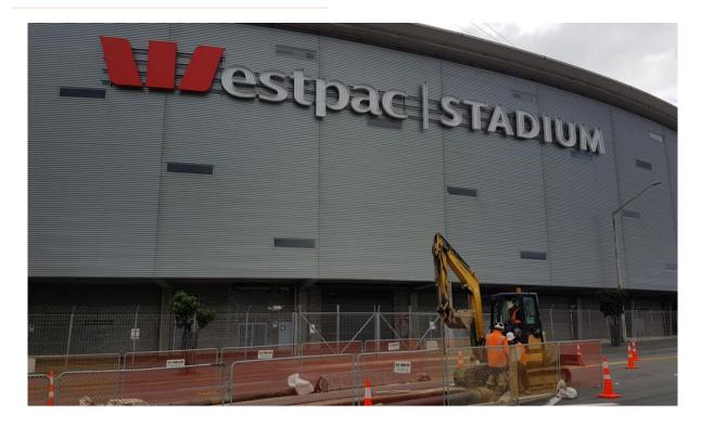
The Waterloo Quay Wastewater renewal was intended to address a poor condition asset that was at the end of it's design life. As part of the work the main was upsized to cope with high flows from the upstream catchment. The proposed solution was to upsize the existing sewer from a 150mm diameter earthenware main to a 250mm OD PE100 main by pipe bursting. The existing main was approximately 2.5m deep in the carriageway of Waterloo Quay with a section under the rail crossing into Centerport.
