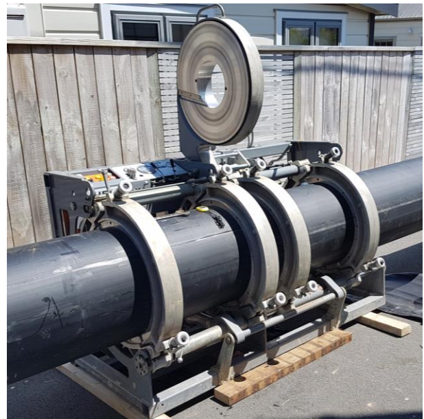
560OD PE100 SDR17 being butt fusion welded
