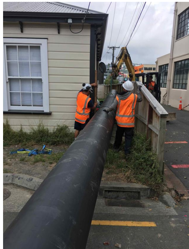
Lindin, Tom & Gerry manoeuvring the new pipe around a neighbouring property
